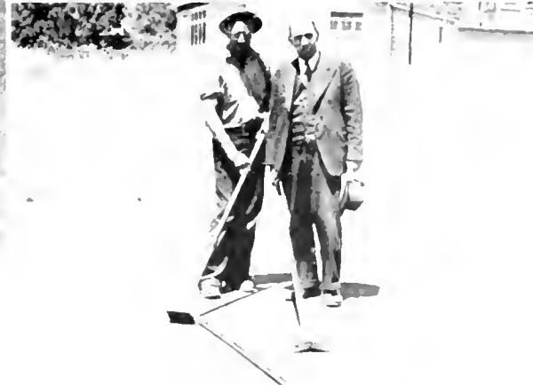
1—Durable, raised bars of asphalt concrete instead of plant-mixed bars placed in advance of safety zones adjacent to street-car tracks by use of plywood forms that rendered unnecessary the building of barricades needed to protect plant mix bars while curing. 2—Shaping iron on tracks in form. 3—Tamping iron for shape in ends of bars. 4—City Engineer Klassen of Daly City, who devised method, and equipment operator Cafferreta.
